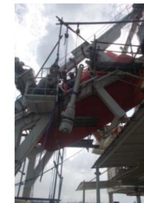
Lifeboat Davit (FF) electric jack replacement in anchorage.
